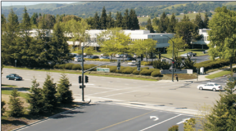
Bishop Ranch 2 as viewed from Bishop Ranch 3 parking structure.
